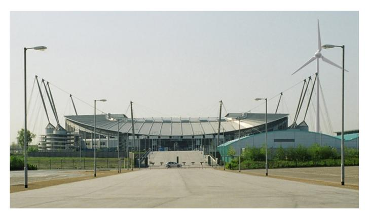
Instead, the football club has incorporated a range of more modest energy systems to lower emissions. Trigeneration systems, absorption chillers, combined heat & power systems (CHP) all help to export electricity internally and externally to the grid.
